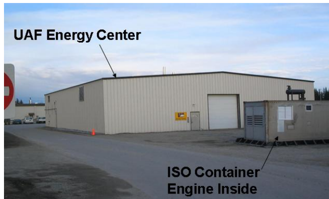
Figure 1 Diesel Generator Location
